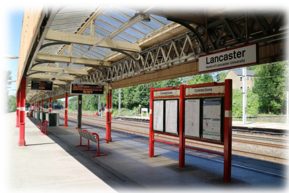
Lancaster Railway Station Platform
